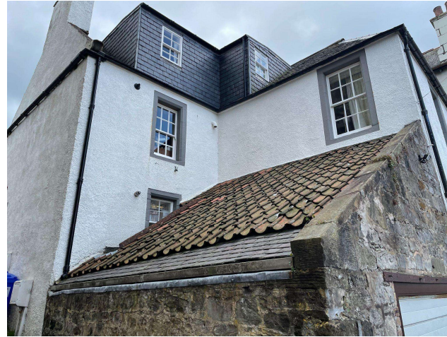
Rear of 56 High Street.
